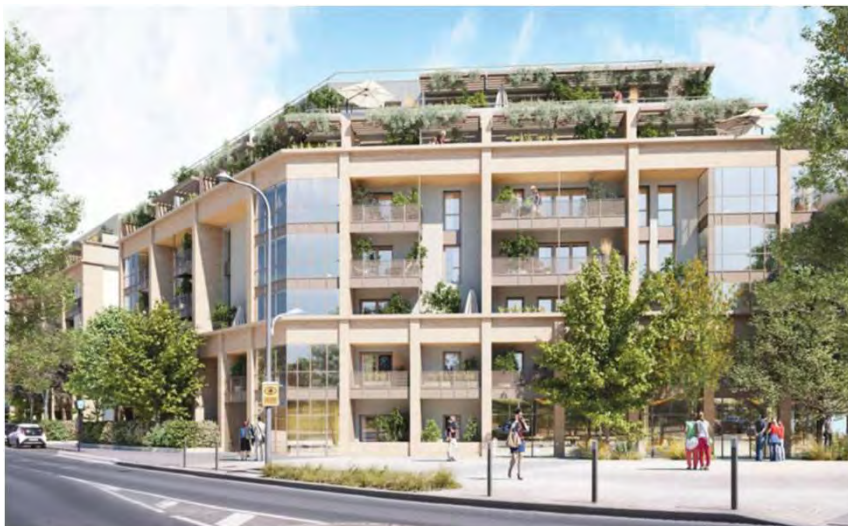
Meudon, 69 intermediate housing units
