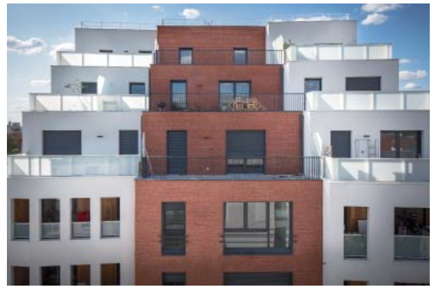
Contracting authority: in'li Construction company: Angevin Île-de-France Architect: Petitdidier Prioux Architectes
